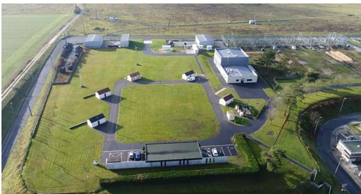
EDF's Concept Grid Network reproduced the installation of the Lérins Islands on a 1/4 scale
